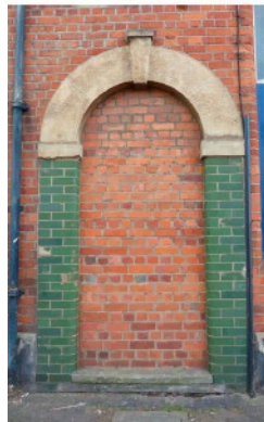
Existing green glazed brick used
