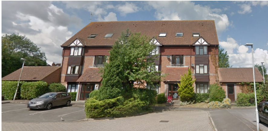
Image of the former block (Google Street View, 2019)
